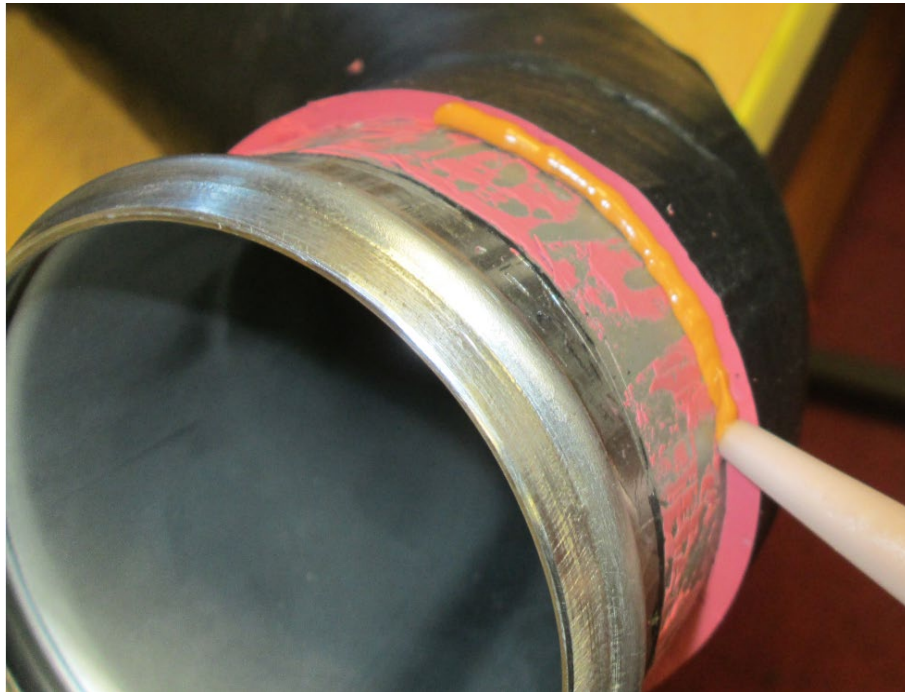
Figure 18 – Application of High Temperature Silicon
