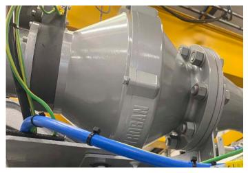
Air inlet shut-off valve and air inlet flame arrestor
