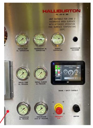
A colour touchscreen HMI (Human Machine Interface) displays the current safety status and the diesel engine control and monitoring screens can also be integrated. For example equipment controls, pump sensors, as well as fire and smoke detectors can all be fed into Ex-SCS.
